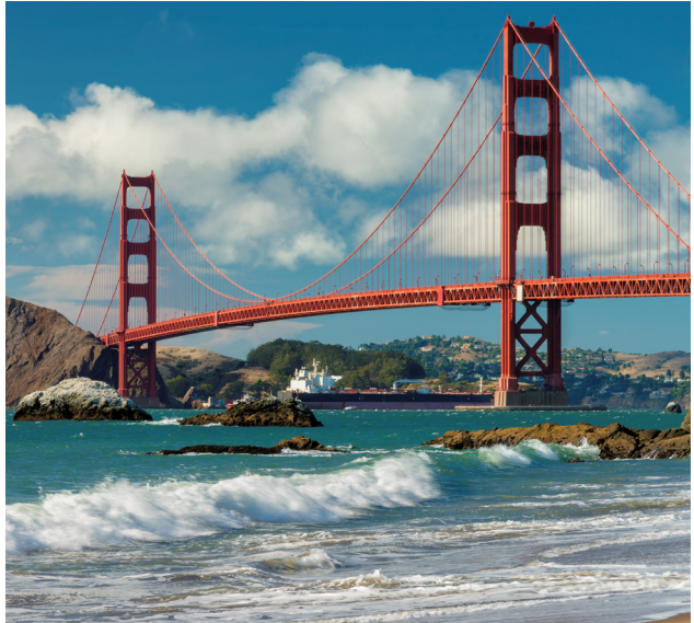
Golden Gate Bridge in San Francisco, California
