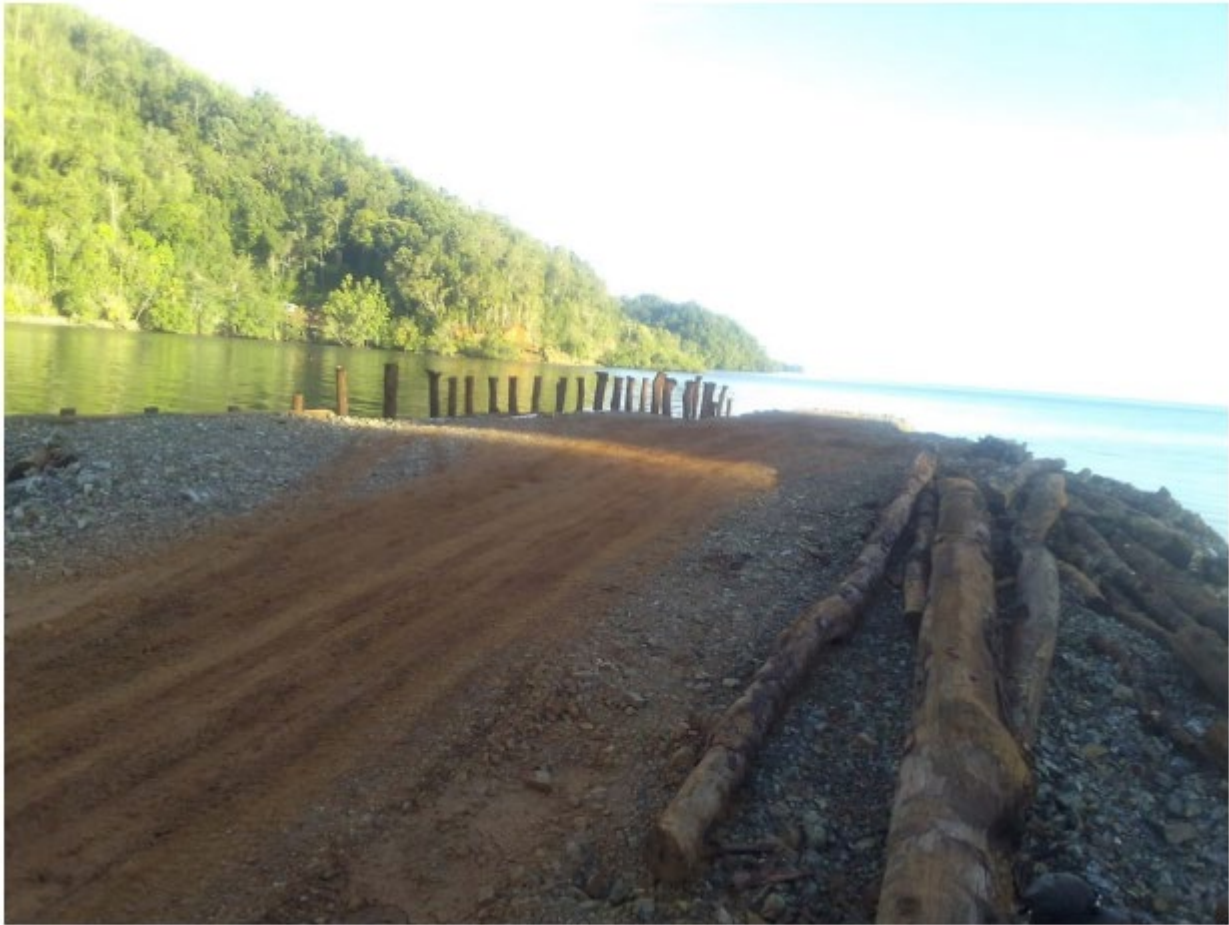
Photo 1: Construction of eastern face of DSO Loadout Wharf nearing completion.
